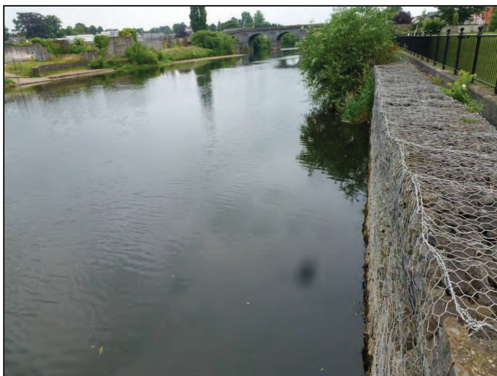
Plate 4 Gabions occur along left bank of the River Nore within the study area.
