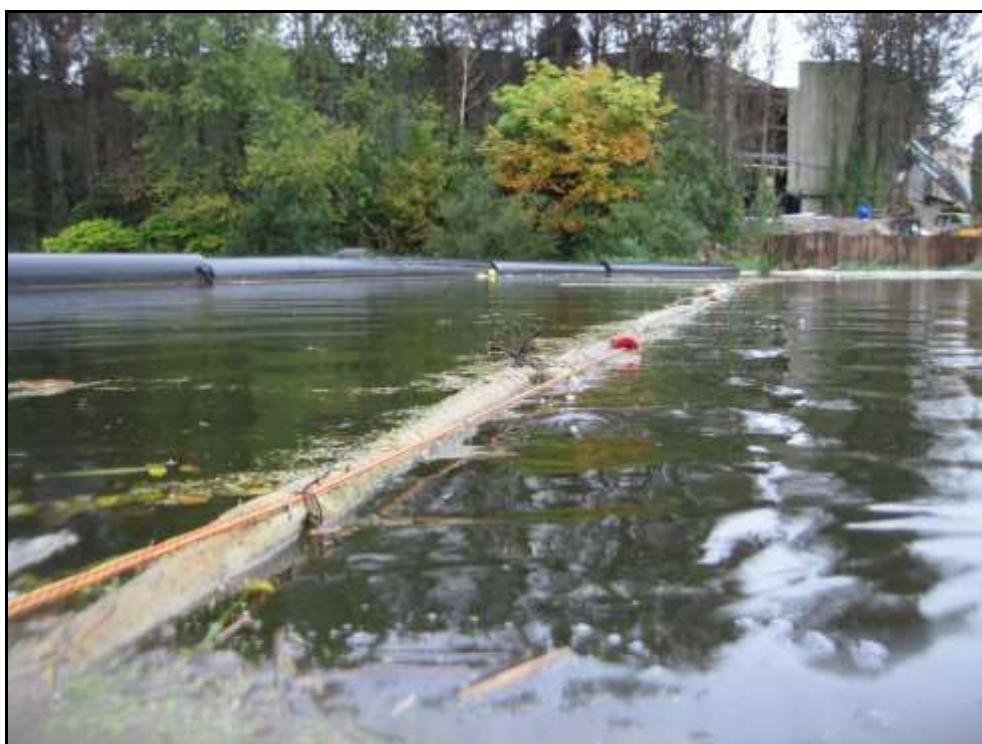
Plate 4 Boom positioned across the river downstream of the works.
