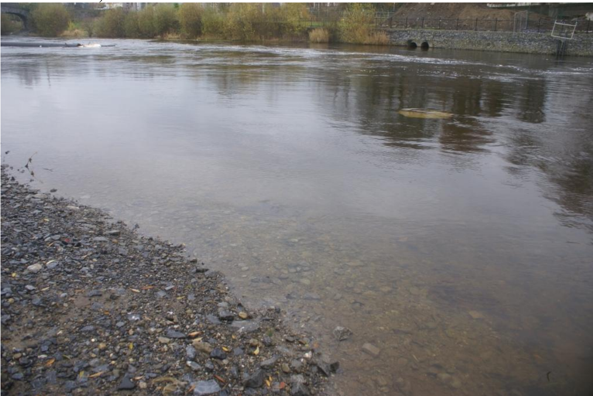
Photo 2: Site 2, At Construction Site
