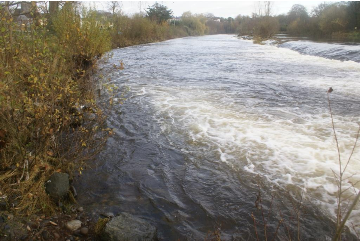
Photo 4: Site 4, Downstream of Weir
